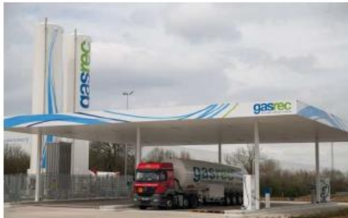
LCNG station, Gasrec, UK
