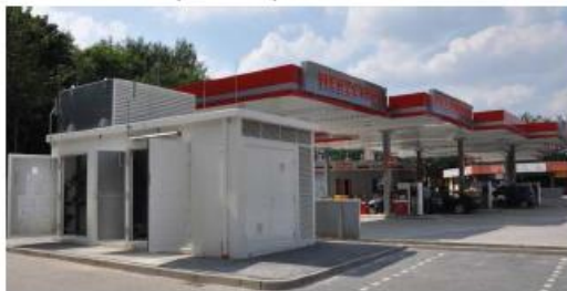
CNG station, Bohlen & Doyen, Germany
